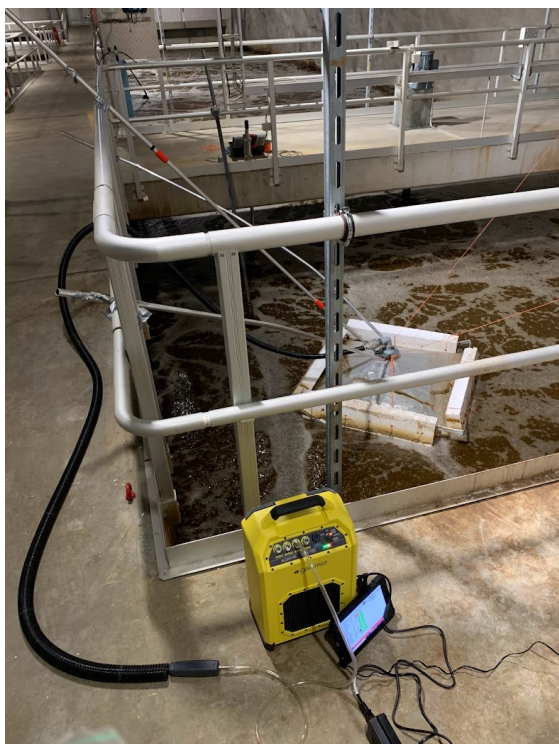
(a) Setup at Kakolanmäki WWTP.
